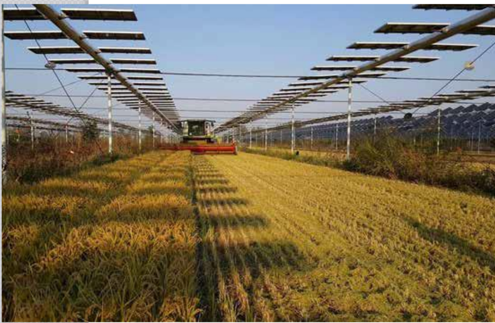
System with high mounting structure and narrow PV modules.
